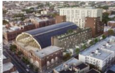
A rendering of the Bedford-Union Armory redevelopment with added apartments and condominiums.
